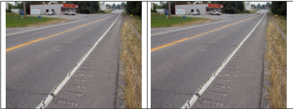
Example of rumble strips placed on a shoulderless roadway, Arch Street Pike in southwestern Little Rock
